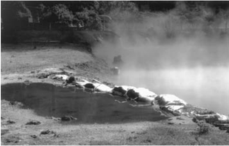
Photo 2. Geothermal brine discharged over the rim of the evaporation pond of the Az-2 well unit during July and August 1995. Damages from this, such as landslides and fractures on the rim and the exterior part of the wall, were provisionally sealed with sand bags.
