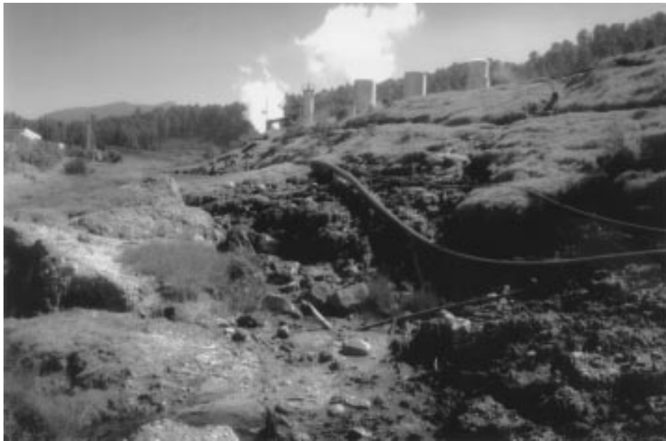
Photo 1. Fractures and permeable material of the pond wall (right side of the photo) of the leaking Az-22 pond (production towers and evaporation pond of the Az-22 unit in the background) cause the spill of oxidized geothermal brine into the adjacent stream (river course from the upper left part of the photo towards the lower, central part).
